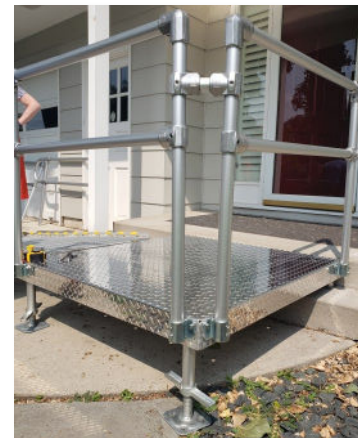
Secure Ramp-to-Platform Connection Ramp may be lifted up for use elsewhere.
